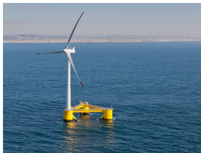
Fig. 1.8: Floating offshore turbine from Kincardine Offshore Floating Wind Farms in Scotland (Cobra Group, 2019)
