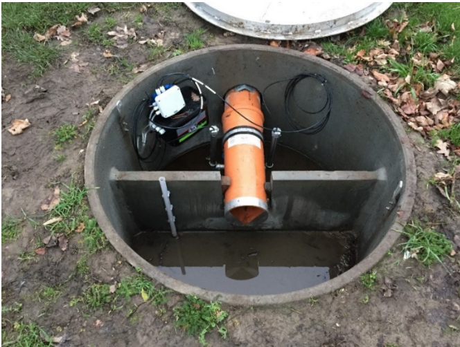
Figure 2.7. Flow-meter manhole with a V-notch weir.
