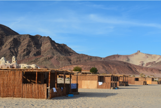
Figure 2. Sample for the hut design using bamboo reeds and local wood.
