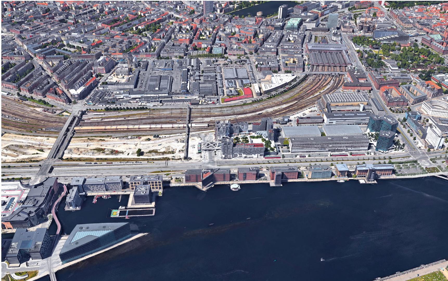
Fig. 5: Kalvebod Brygge development in Copenhagen. (Google earth)
