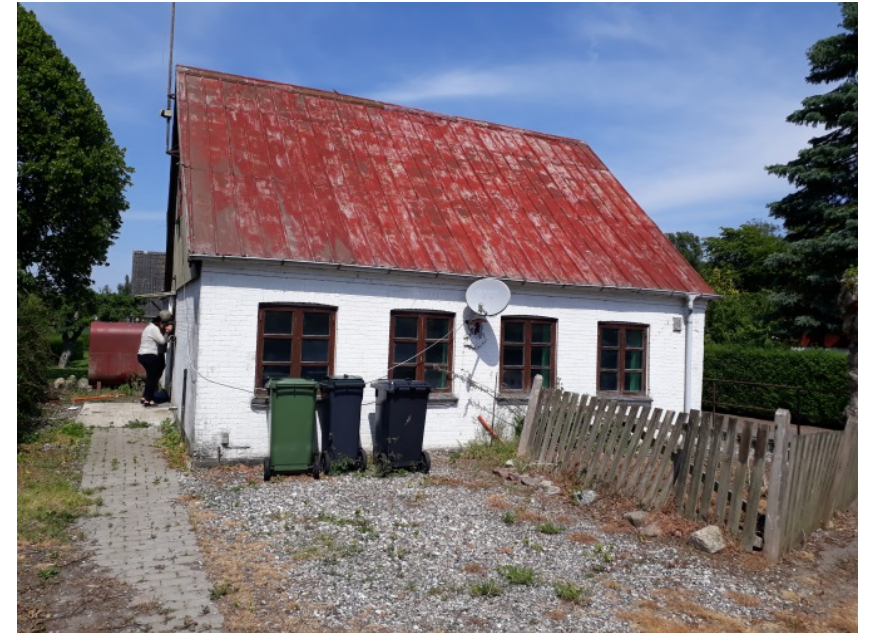
Private renting of a derelict single-family house, municipality of Lolland. The municipality has condemned the house, but it is believed to be rented out still. Heat and electricity is disconnected. The owner bought just before GFC in 2006, has a debt on 30.000€ in the house, impossible to sell for this price today. Too expensive for the municipality to buy and demolish. Owner hope to get some of his money back by renting out the house to low-income families.
