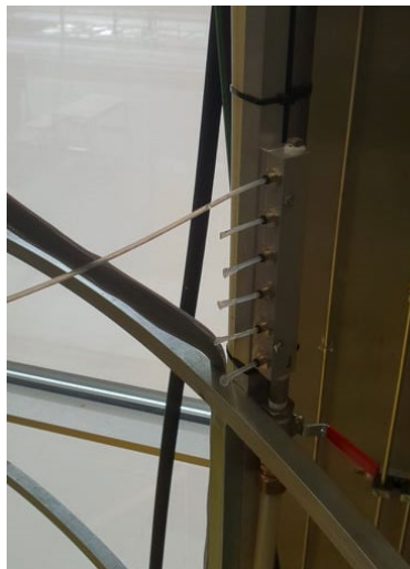
Fig. 3.14. The vacuum access point on the working platform
