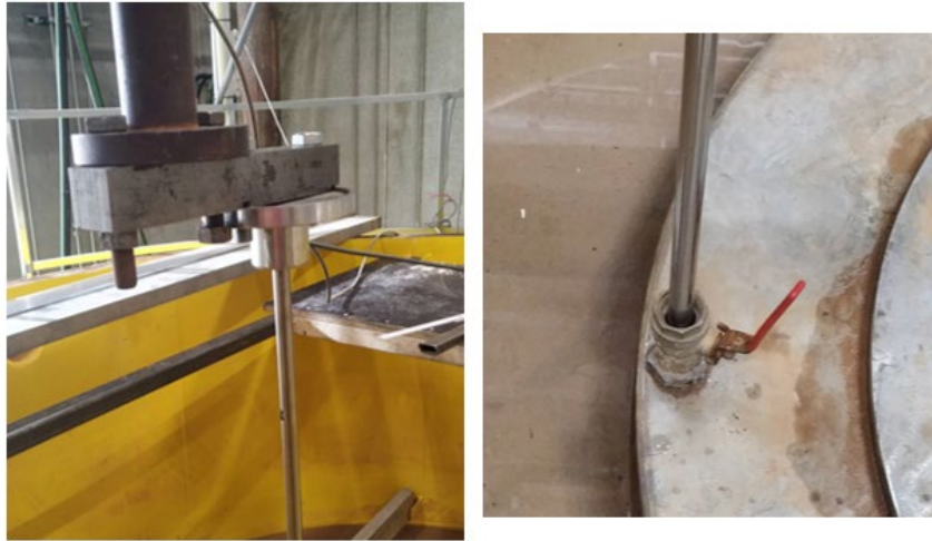
Fig. 4.10. CPT performed with extension piece; CPT inside the valve
