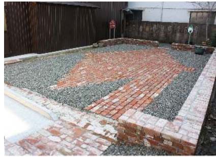
Figure 8: Finished brick bench park
