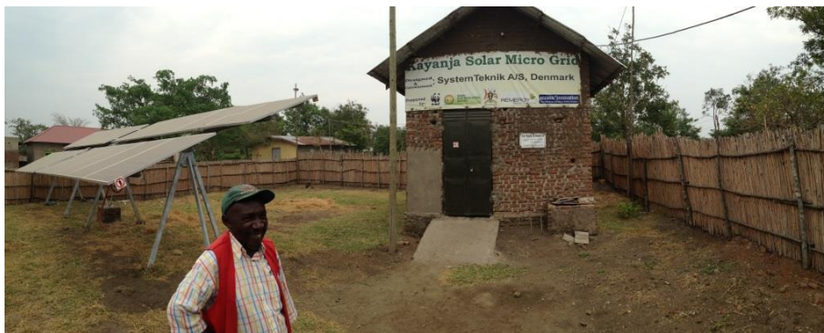
Figure 11 – The Remergy electrical micro-grid installation in Kayanja, Uganda (Vandenbroeck, 2015).
