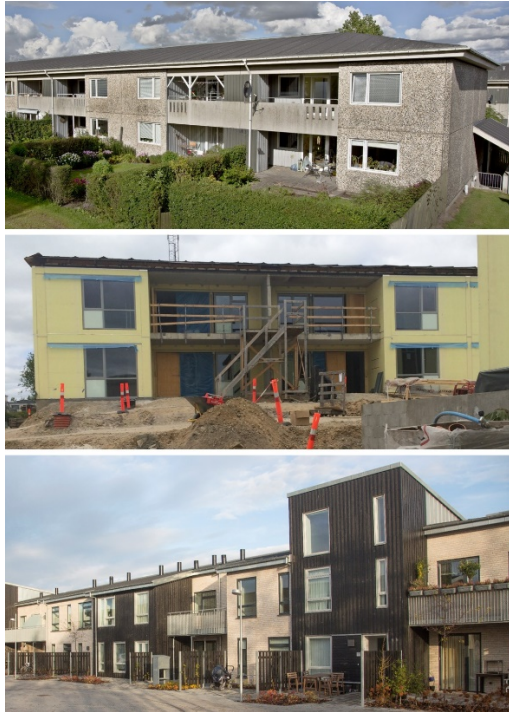
Figure 6: The case building before, during and after renovation.
