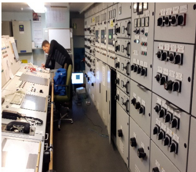
(b) Engine room
