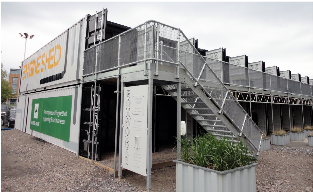
Figure 36: Box Works, Plot 6 Temple Quay
