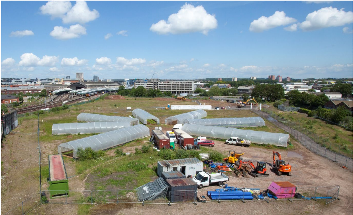
Figure 35: The Severn Project, Former Diesel Depot Site
