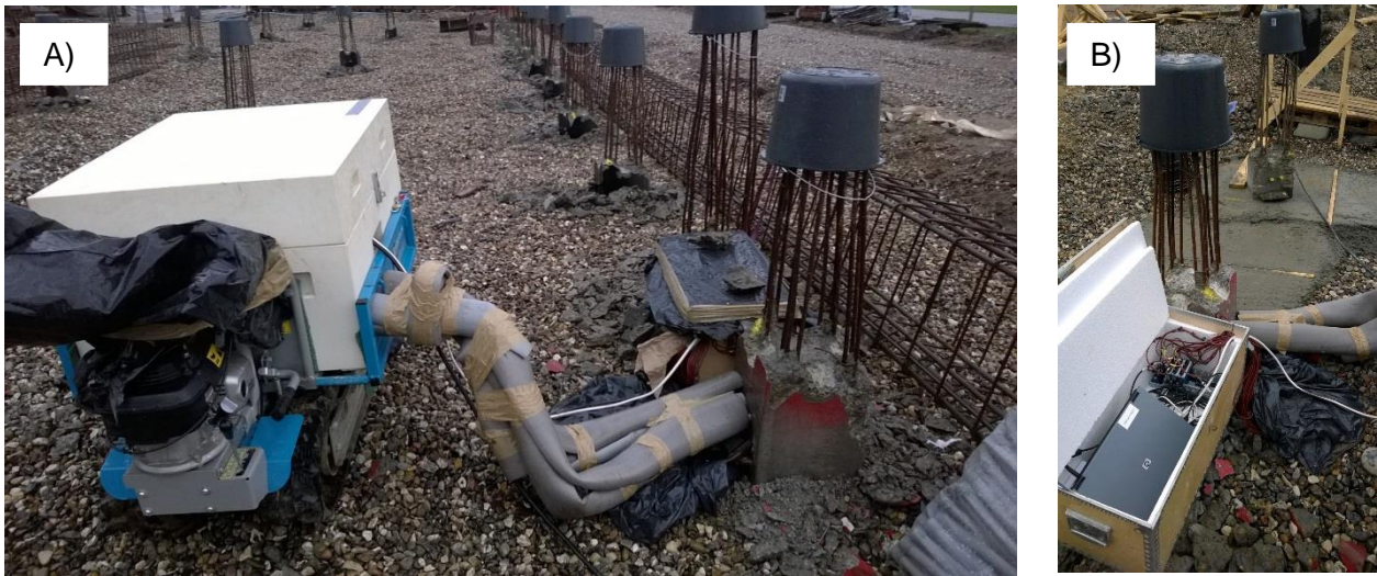
Figure 21: A) Ongoing TRT of the 16 m long EP at Rosborg North. Inlet- and outlet pipes are insulated to prevent disturbances from ambient conditions. B) The adjacent box, covered with black plastic bags contains the computer and the modules to log the temperature data from the Pt100 temperature sensors casted into the pile (see Figures 11 and 20).
