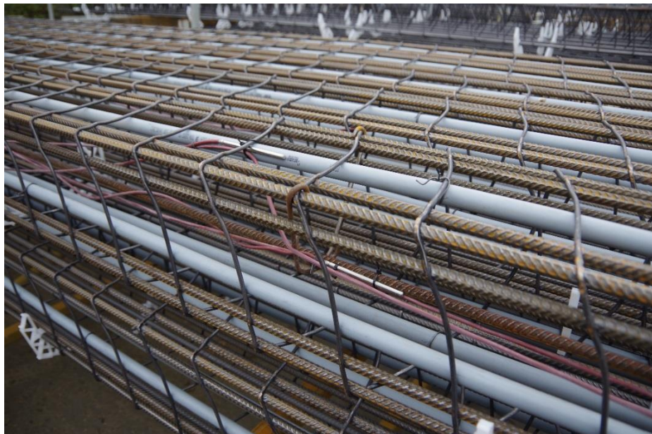
Figure 20: Pile instrumentation with Pt100 temperature sensors.
