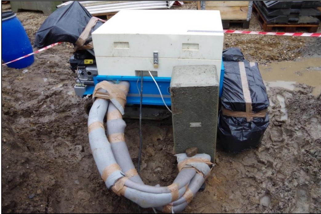
Figure 18: Ongoing TRT of the 18 m long EP3 at Langmarksvej. Inlet- and outlet pipes are insulated to prevent disturbances from ambient temperature conditions. The adjacent box, covered with black plastic bags, contains the computer and the modules to log the temperature data from the underground Pt100 TSA.
