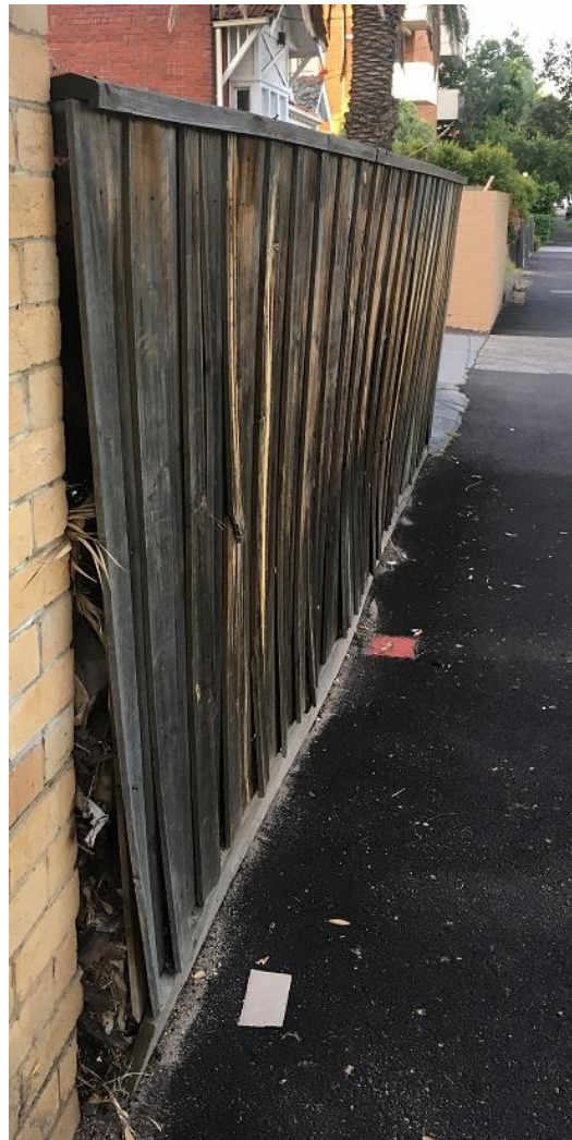
Figure 3. Practical issues of ambiguity as to the limits of boundary occupation. At the few cm level, this fence exhibits: (a) an offset from an abutting boundary on the same alignment; (b) non-verticality; (c) lack of horizontal straightness; and (d) a somewhat rough and ambiguous surface. (Melbourne, Victoria)
