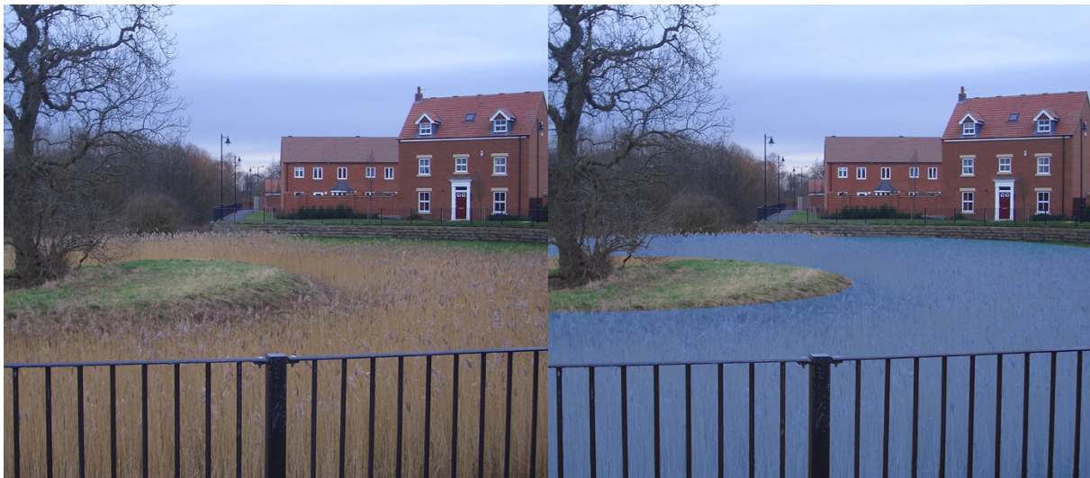
Figure 10: The Great Park Development, UK has green natural spaces that are designed flood with excessive storm water.
