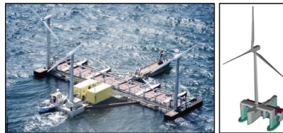
Figure 1. Left: The P37 prototype during sea testing in the Danish sea. Right: Conceptual drawing of the P60/P80 device considered in the present study ( Floating Power Plant , 2015).
