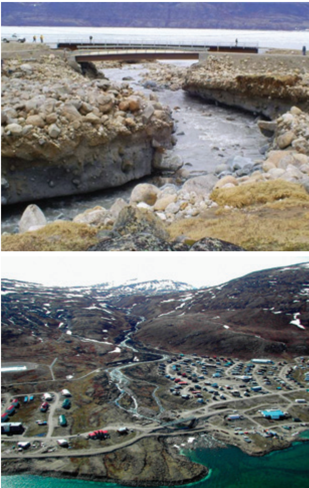
Figure 10.26 Extreme peak discharge of the Duval River in June 2008 resulted in downcutting of the riverbed, generating thermo-erosion and causing terrain collapse and the destruction of the Pangnirtung bridges (from Gosselin, 2013, and Carbonneau, 2014).
