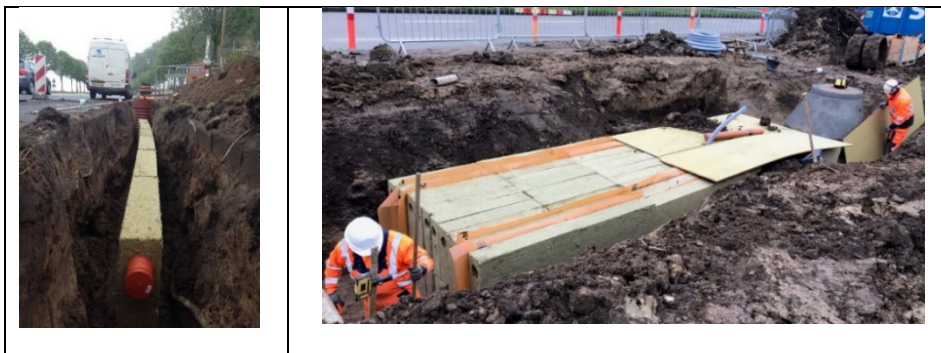
Left: Construction of a pilot-scale filter at Strandvejen
