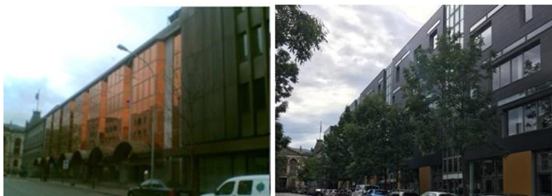
Figure 8.5 Sparebank 1 buildings: the old and new buildings
