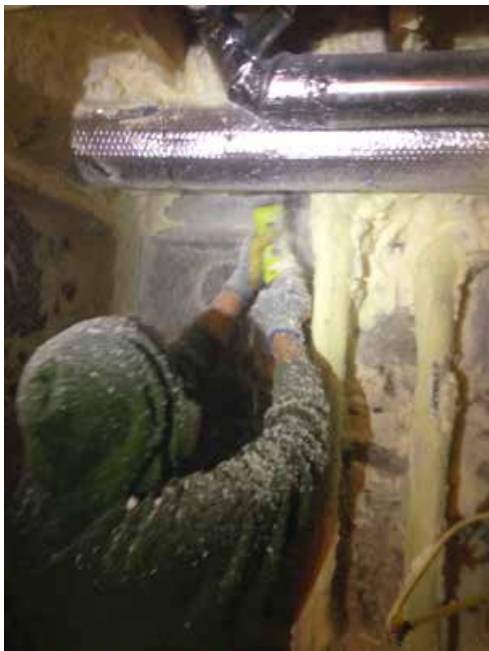
Figure 3.2 Trimming and removal of closed-cell foam using a powered brush tool. Source: Author's own elaboration
