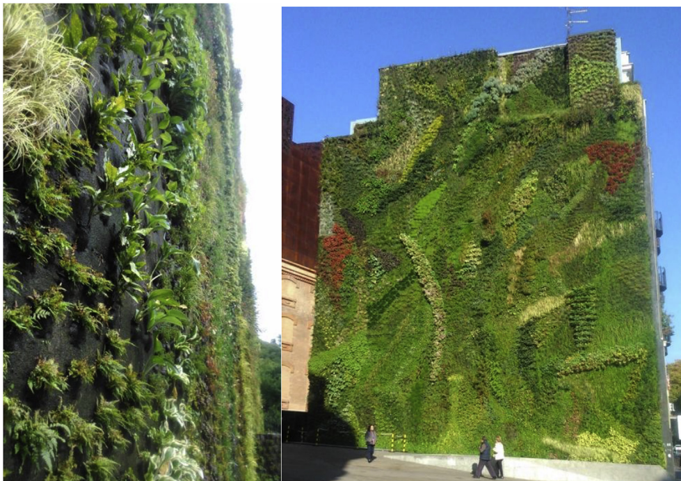
Fig. 1. Green wall installation (Wall 1) at the Caixa Fórum Museum, Madrid, Spain.
