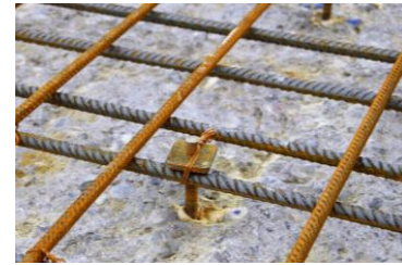
Figure 7. Bridge rehabilitation with threaded rod and plate
