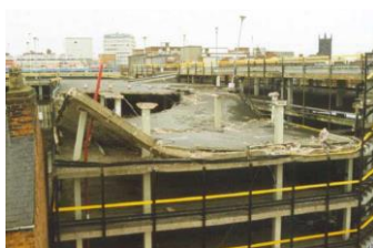
Fig. 12. Accidents due to punching shear: Wolverhampton (l), Gretzenbach (r)
