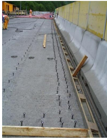
Figure 11. Bridge rehabilitation with optimized Connector HCC
