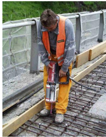
Figure 11. Bridge rehabilitation with optimized Connector HCC
