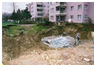
Fig. 12. Accidents due to punching shear: Wolverhampton (l), Gretzenbach (r)
