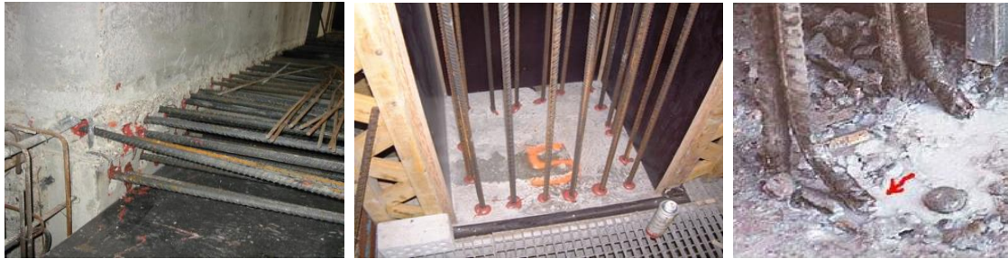
Figure 1. Typical applications of post-installed reinforcement connections
