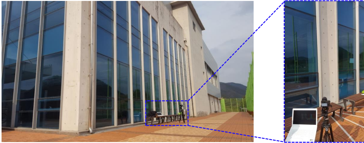
Fig. 5.8 Experimental validation of the proposed approach applied to a concrete wall.
