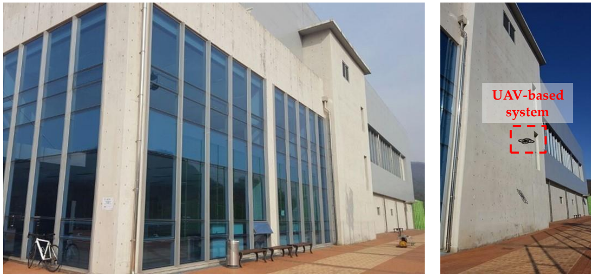
Fig. 4.13 Experimental validation using concrete wall.
