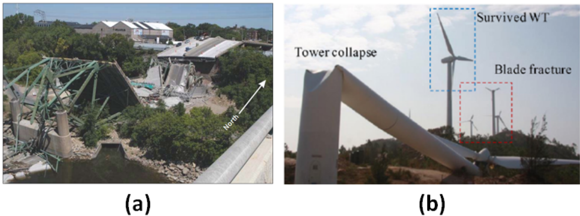
Figure 1.1: Fatigue failures (a) I-35 bridge collapse, (b) a wind turbine collapse
