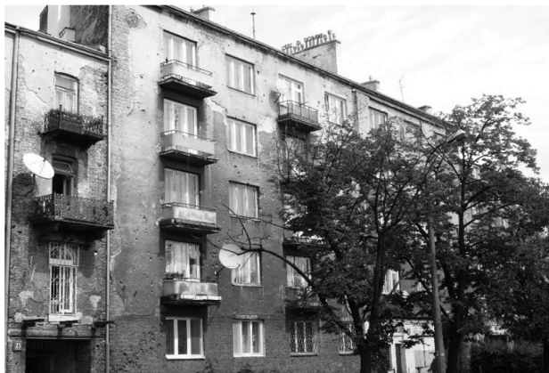
Fig. 1. View of the eastern facade of the building
