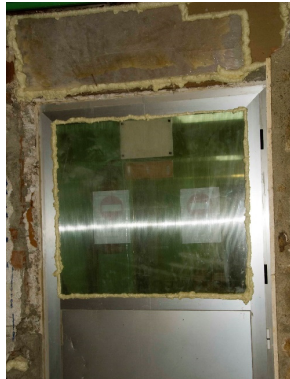
Fig. 1. Biosecurity barrier installed on a hospital site
