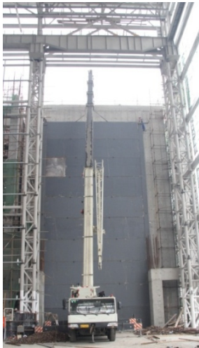
Fig. 5. Construction photo of the door
