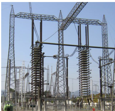
Fig. 1. Steel frame of converter station
