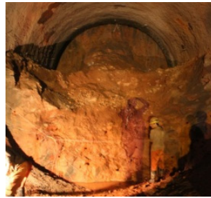
c) Field construction
