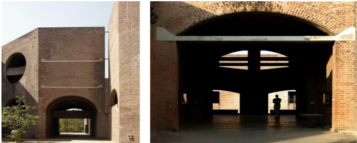
FIGURE 3.1.1: The Indian Institute of Management by Louis Khan displays strong visual expression of material and structure
