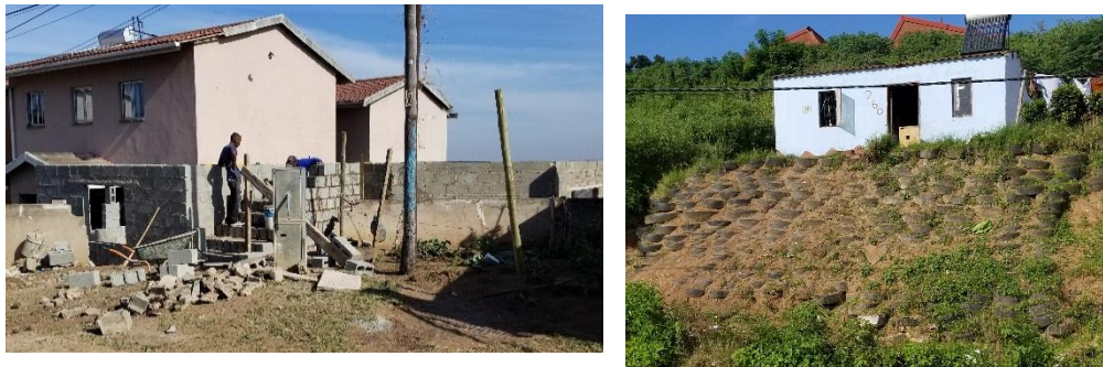
FIGURE 5.1.7: Construction in Welbedacht showing innovation use of materials. (photo by author, 2018)
