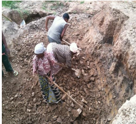
FIGURE 4.2.6 future users involved in construction https://livinspace.net
