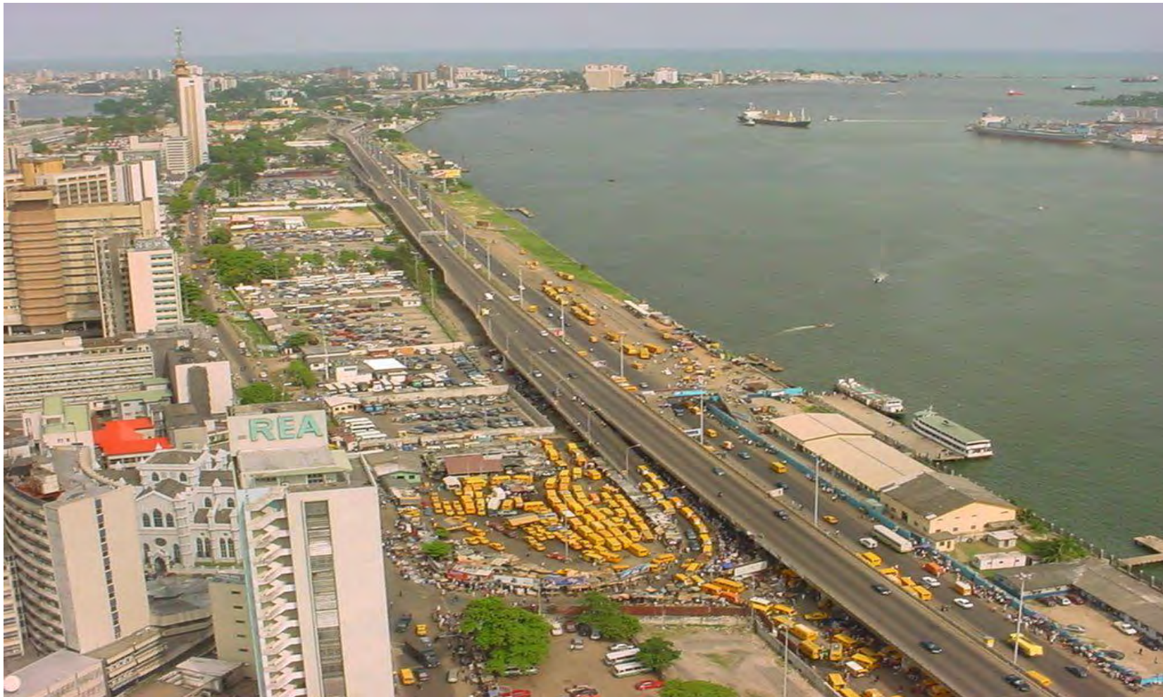
Plate 9.6: Aerial view of the Lagos Island Central Business District, Marina - commercial high-rise buildings and underutilized spaces used as car parks Source: Lagos State Government, Ministry of Information and Strategy 2009 in Filani, 2012
