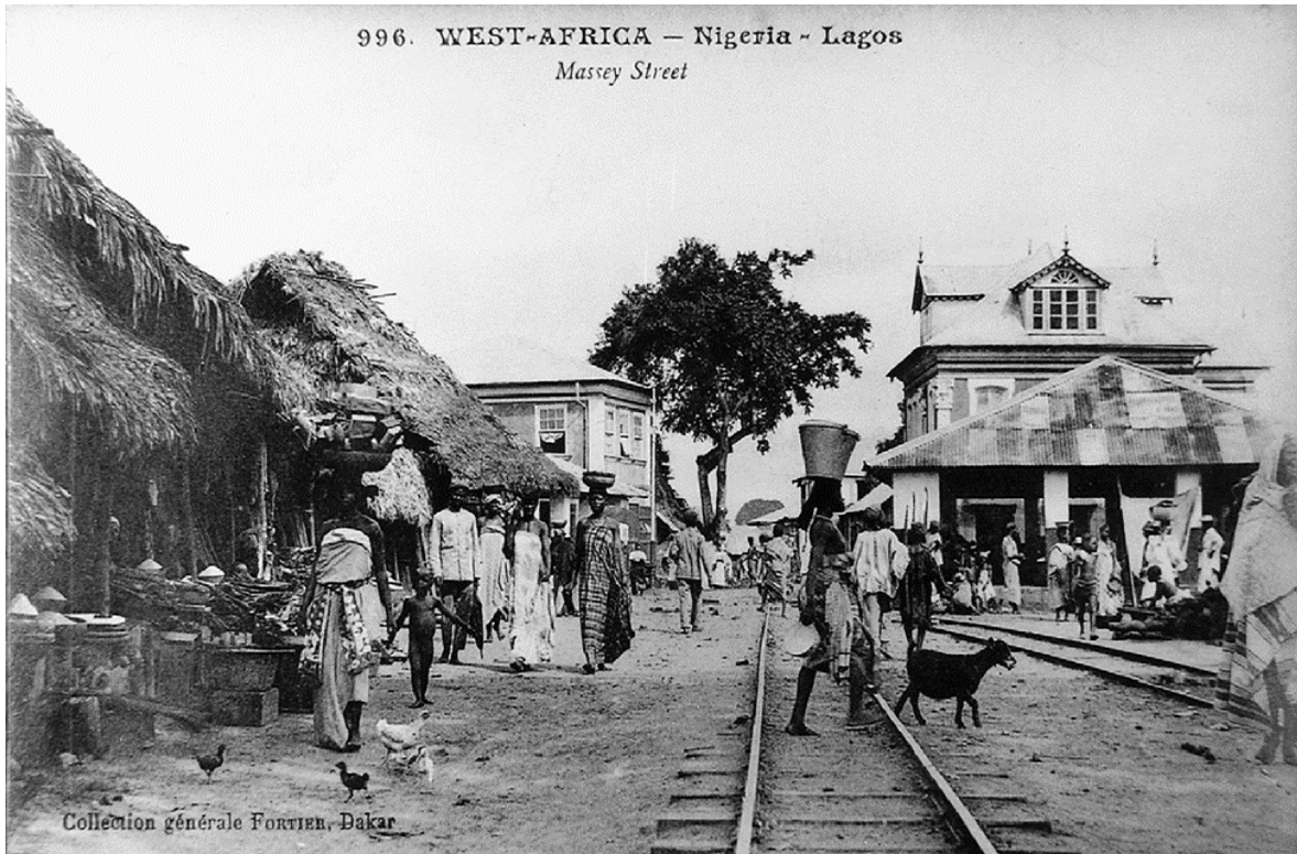
Plate 8.2: Sectoral Development on Massey Street, Lagos Island
