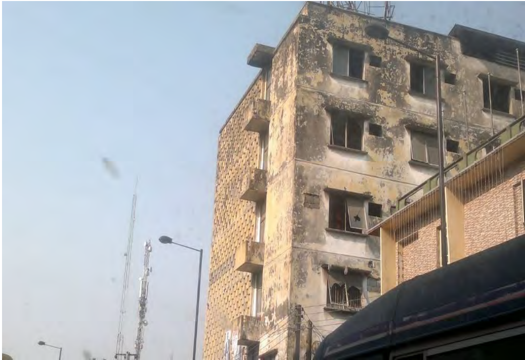
Plate 9.13: Dilapidated building in Lagos Island Source: Author, 2018
