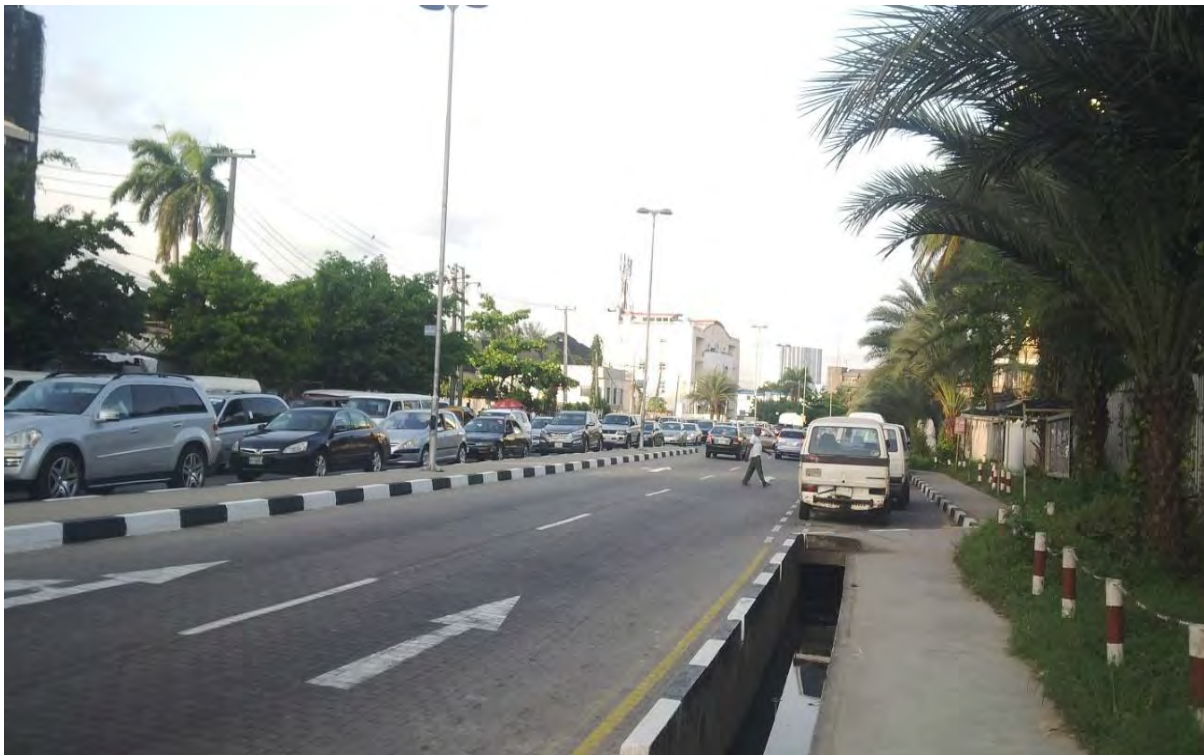
Plate 9.34: Unsafe pedestrian paths over open drainage
