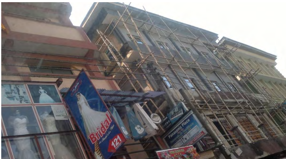
Plate 9.4: Building being transformed for commercial use Source: Author, 2018
