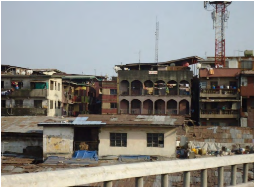
Plate 9.12: Buildings around Idumota, Lagos Island Source: Author, 2018
