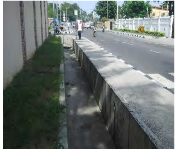
Plate 9.26: Open drainage on Marine Road Source: Author, 2018
