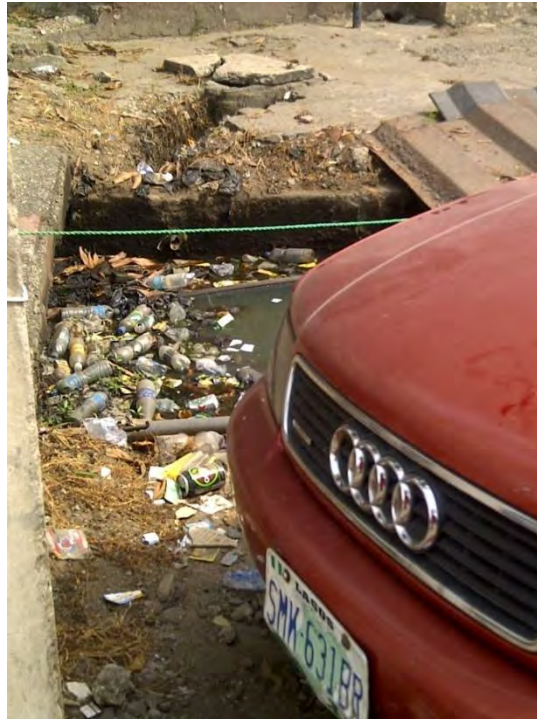
Plate 9.36: A blocked open drain in Victoria Island
