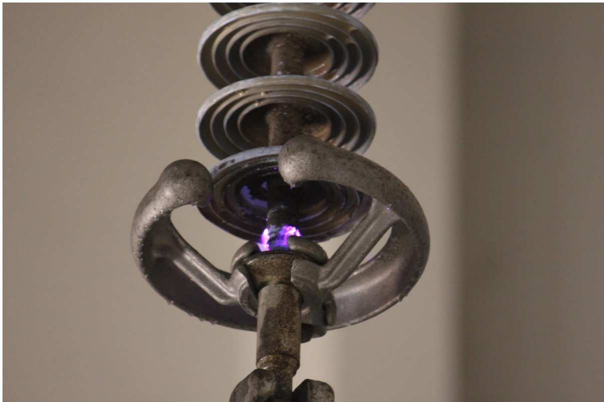
Figure 2-1: Composite insulator, HV Lab (HC) UKZN
