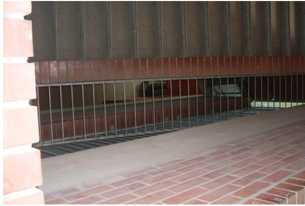
Figure 6.5: A grill between staircases
