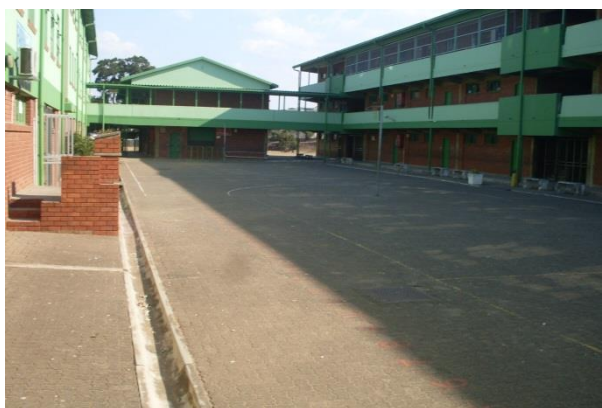
Figure 5.20: The podium and quad area where assemblies are held
