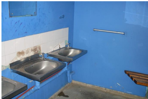
Figure 5.14: Inside the girls' lavatory
