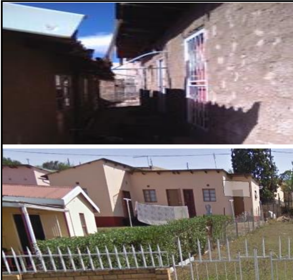
Plate 5.6: Example of backyard structures with safety features
