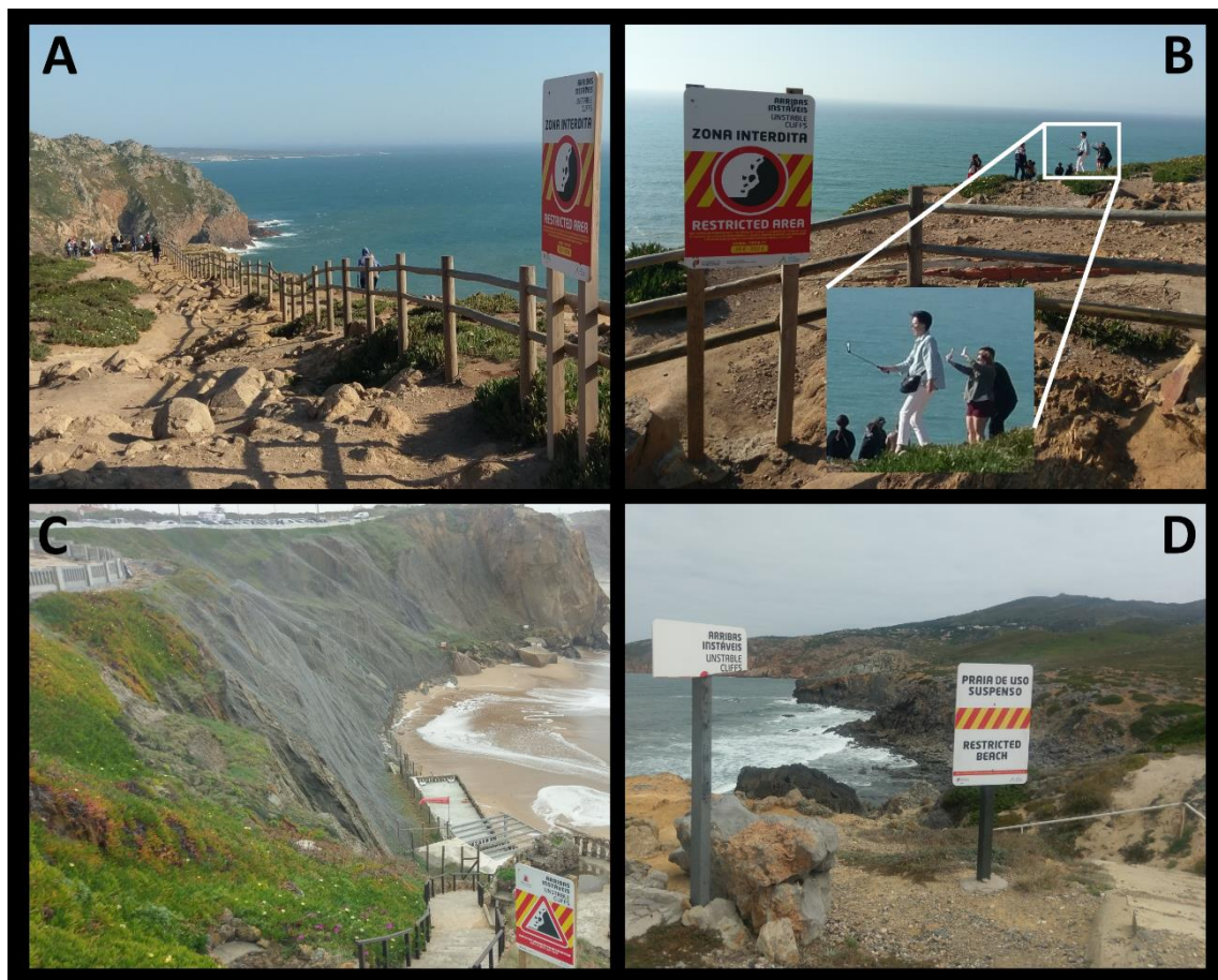
Figure IV.2.1.34. Signalling preventing the occupation of areas at risk in cliff and beach areas, and cliffs' instability. Locations: A and B – Cabo da Roca; C – Praia Formosa, Santa Cruz; D – Praia do Abano, Guincho. Source: Author. Fieldwork April – July 2018.
