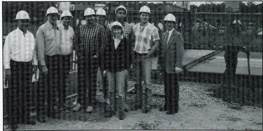
Special Projects Office staffers and members of the Sunset Review team observed a concrete pour in Austin as part of their examination of department operations.
