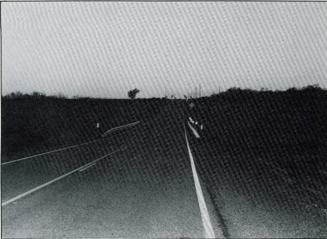
The wide open spaces of the Childress District translate into many miles of roads, such as this farm-to-market road, to maintain and rehabilitate.
