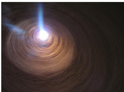
Fig. 1 Left, constructing semicircular domes by increasing the amount of mortar as dome circularly goes higher, Interior View, Meibod Ice House, Yazd, Photo: by Authors, 2007
