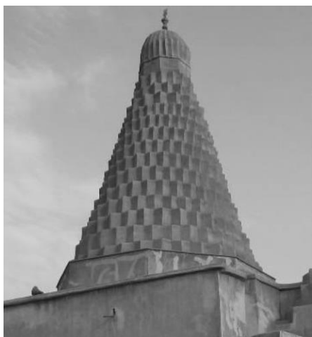
Fig. 4 Left, transmitting loads in Ourchin domes through the change in the form of external shell and in the form of plan [2]
