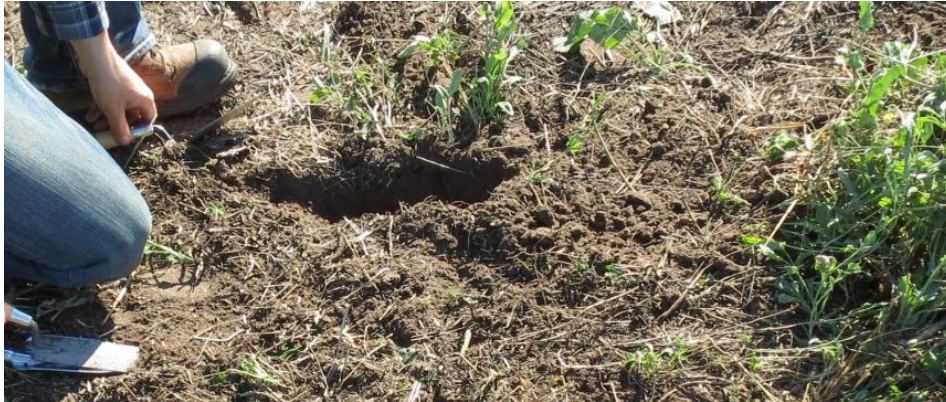
Figure 4.38. Step No. 4: Digging the localization hole.
