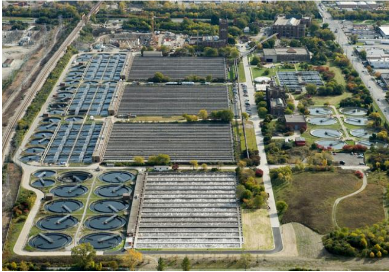
Figure 6: Stickney Water Reclamation Plant [22]
