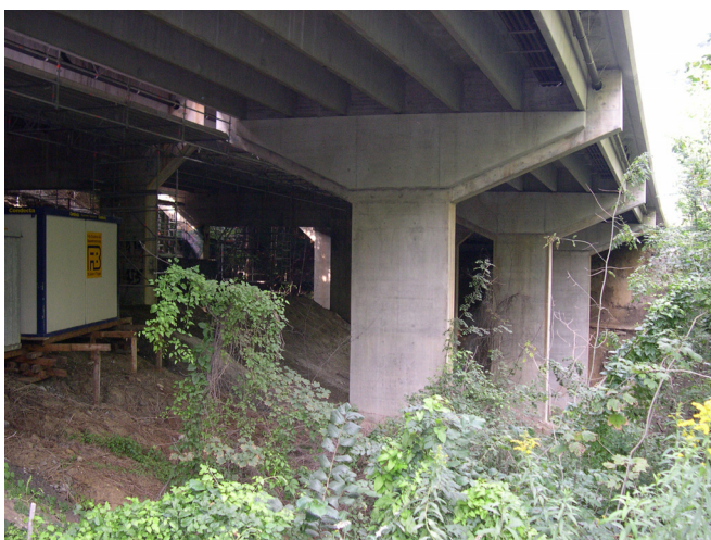
Fig. 2.37: Viadukt Untere Weid on Highway A1 in SG left: View of piers and soffit of precast concrete girders, right: Plan view and elevation
