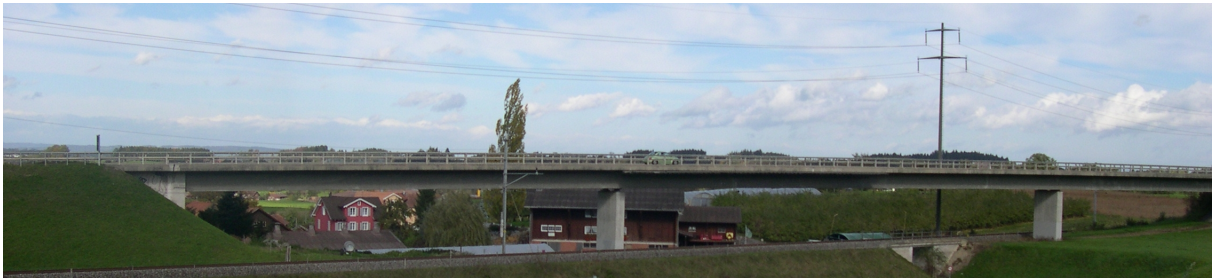
Fig. 2.39: View of bridge over railway on west-bypass Gossau (SG)
