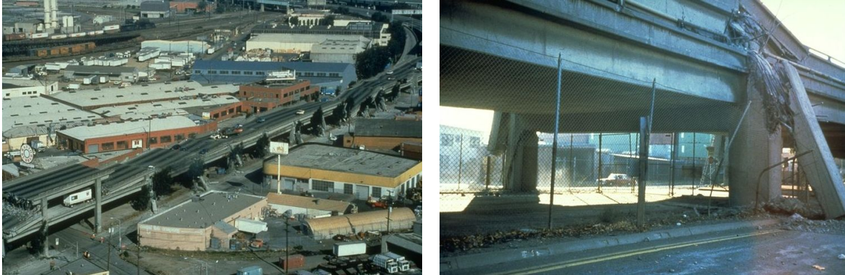
Fig. 2.13: Collapse of the Cypress Viaduct during the Loma Prieta earthquake 1989 (Source: NISEE)
