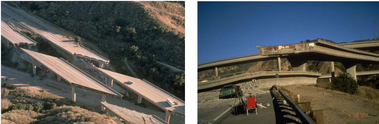
Fig. 2.1: Unseating of superstructure at Interstate 5 during Northridge earthquake 1994 left: Gavin Canyon (Source: NISEE), right: Highway 14 (Source: NISEE)
