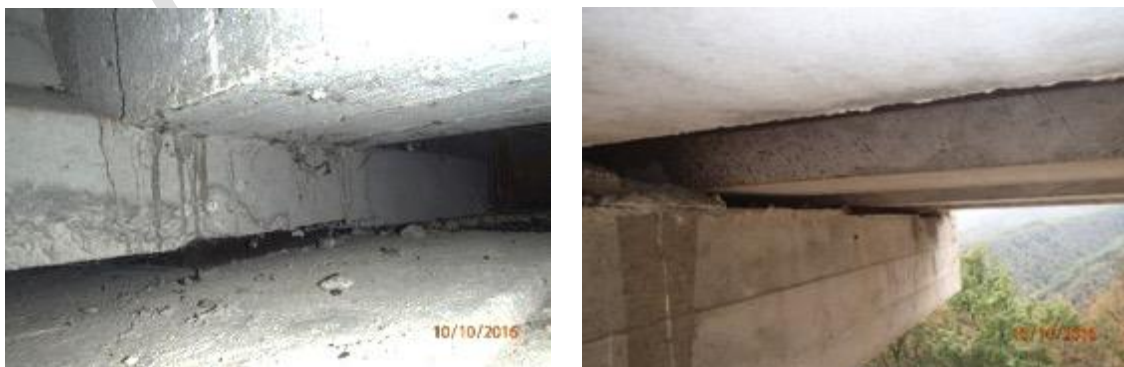
Figure 17 - Bearing pads of a viaduct investigated along SS685 (courtesy of Totaro).
