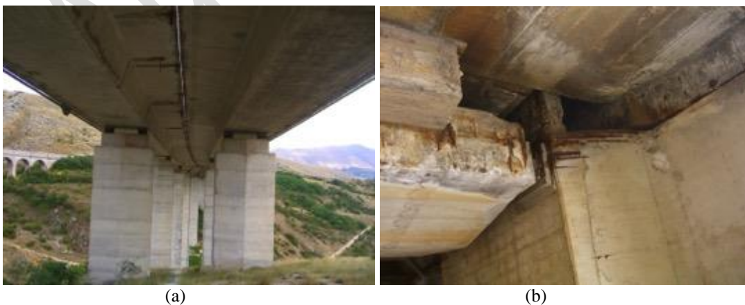
Figure 7 - "Della Valle" bridge along Highway A24, Italy: (a) bridge configuration; (b) typical damage due to lack of maintenance.
