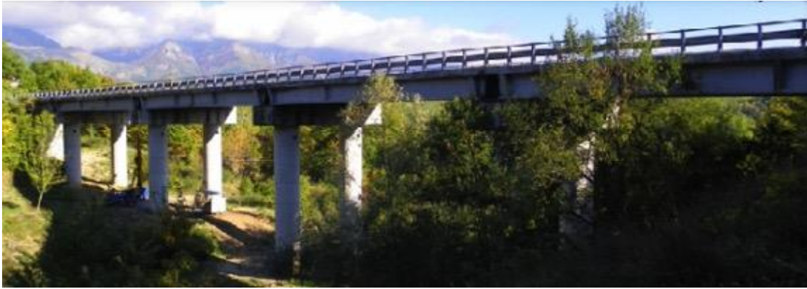
Figure 16 - "Scandarello" reinforced concrete viaduct (42.643309 N, 13.266802 E; adapted from [29]).
