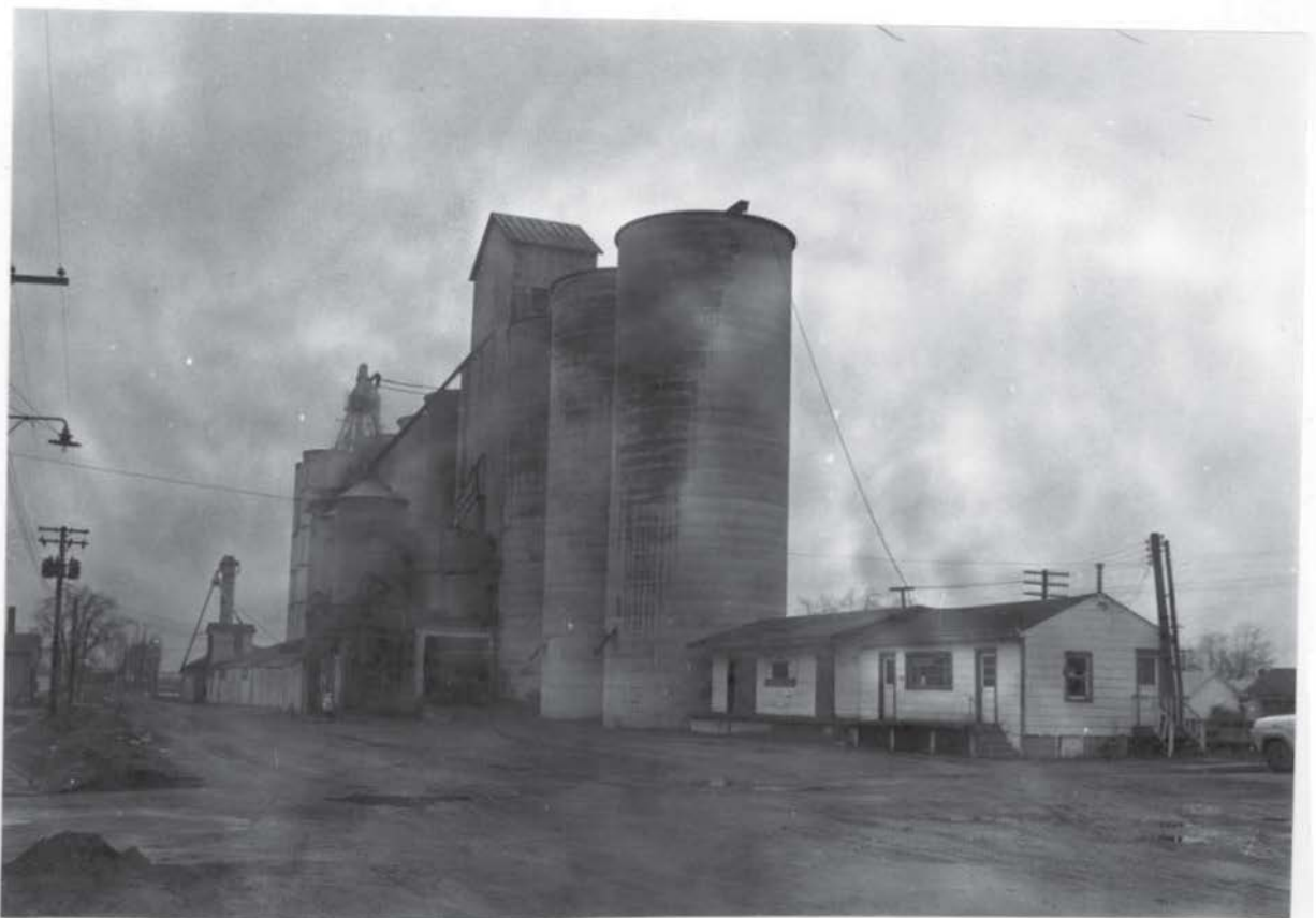
Fig. 3-4.--The concrete silo type of elevator structure. This elevator is located north of the boundary. (Palmer Grain Co.--Palmer, Illinois).
