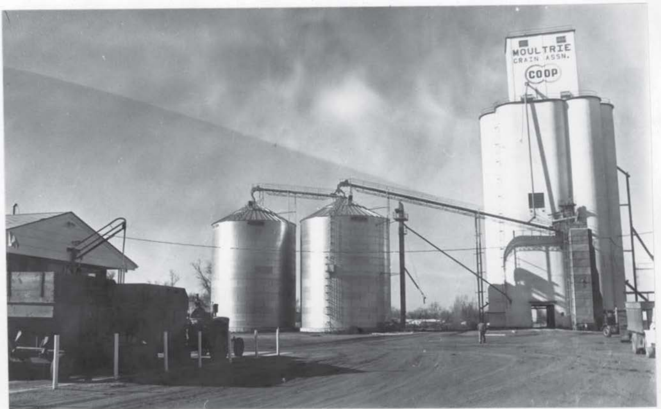
Fig. 3-10.--Expansion of capacity by use of steel bins at elevator located north of the boundary. (Moultrie Grain Assn.--Lovington, Illinois).
