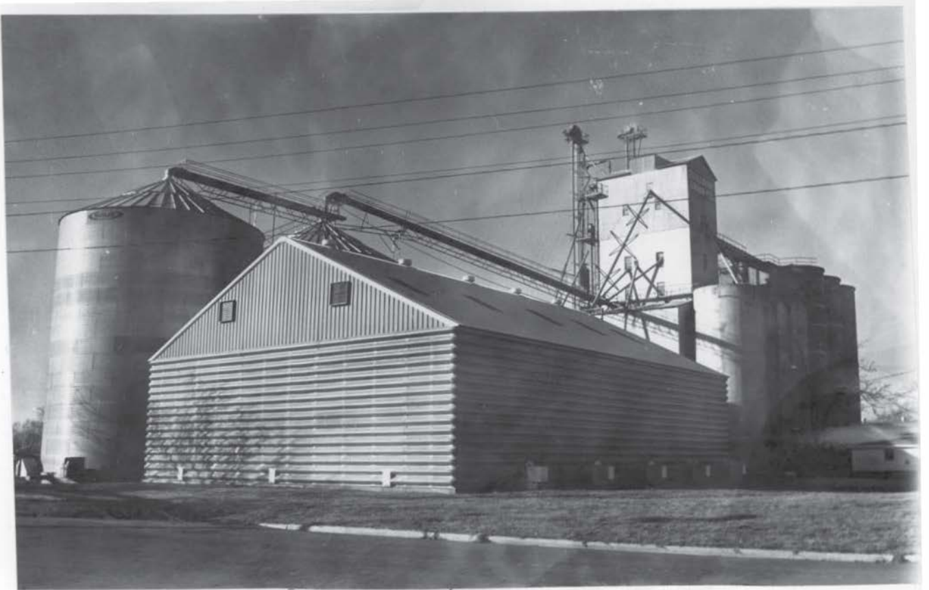
Fig. 3-9.--Expansion of capacity by use of a metal shed used for storing grain. This elevator is located north of the boundary. (Sullivan Grain Co.--Sullivan, Illinois).
