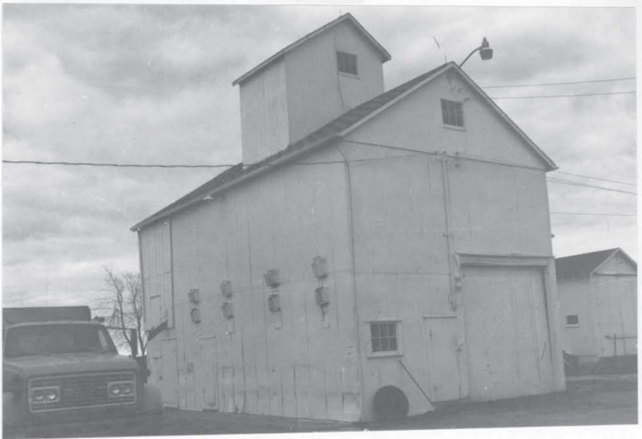
Fig. 3-3.--An example of the wooden building with overhead bins type of elevator structure located south of the boundary. (Rieke Elevator--Nokomis, Illinois).
