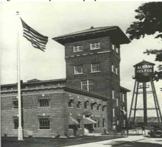
Figure 1: Albany Felt Company 1920's
