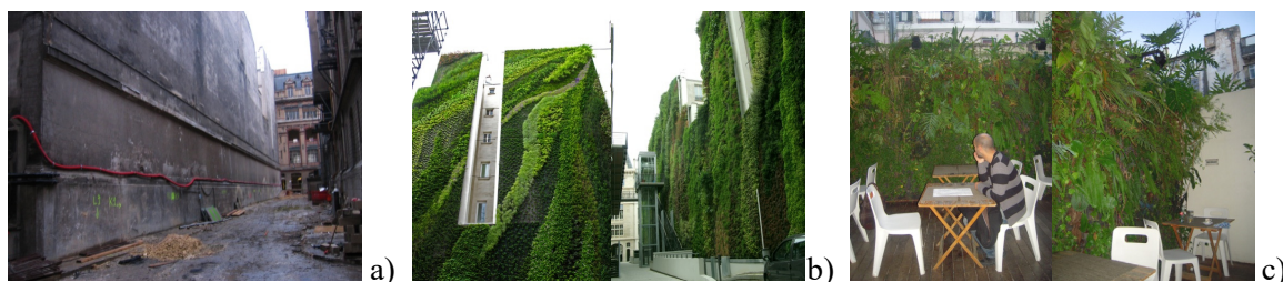
Figure 6. Rue d'Alsace in Paris, France (a) the previous blank wall; (b) the living wall; (c) the inner courtyard of Royale Café in Lisbon, Portugal
