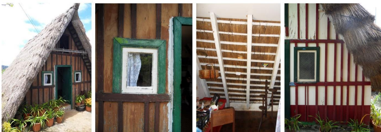
Figure 1. Vernacular houses of Madeira with thatched high-pitched roof and wooden or stonework walls.
