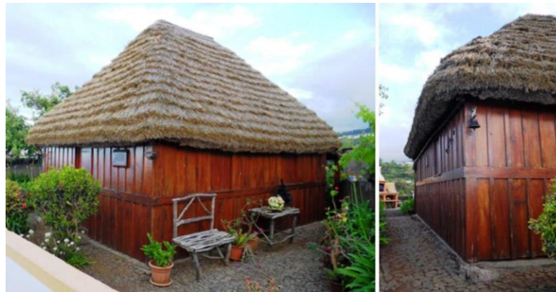
Figure 6. A refurbished traditional “Redonda” house
