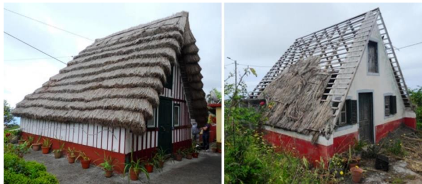
Figure 4. “Meio-Fio” house - Outer view and roof structure
