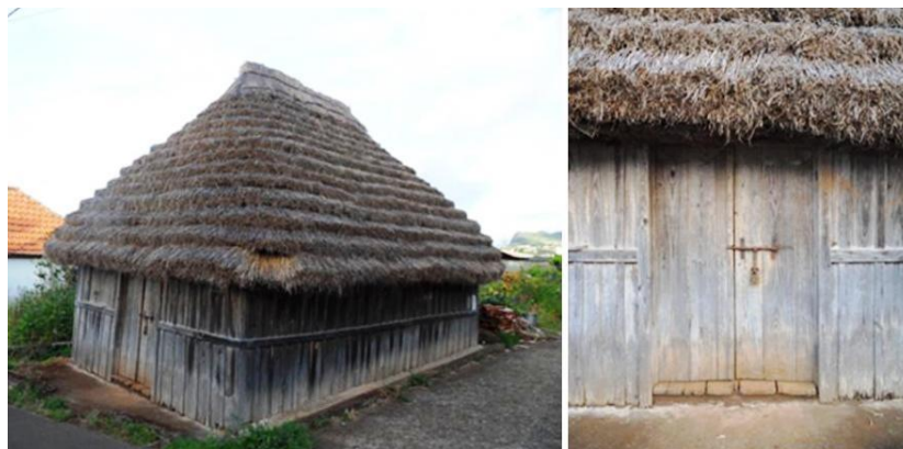
Figure 5. “Redonda” house - Outer view and entrance detail
