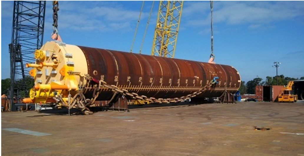
Figure 2.21: Suction pile (image from ref. [30])
