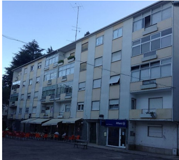
Figure 2. Main facade of the building under study
