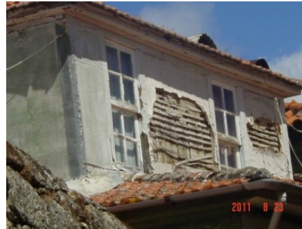
Figure 1: Tabique building and wall.
