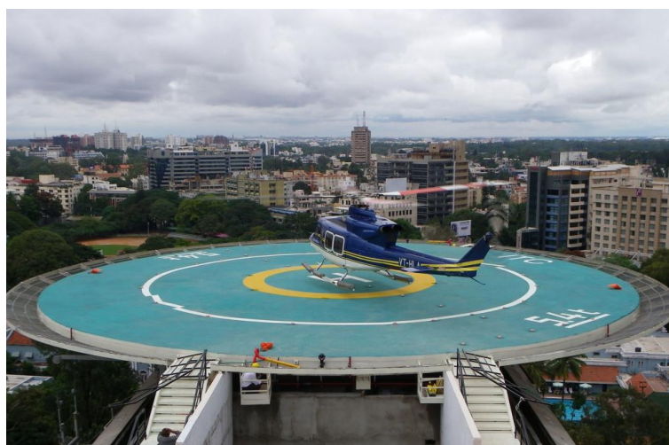
Figure 20 - Markings on Elevated Heliport Platform, Dehli, India, [30].
