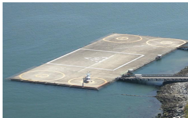
Figure 18 - Surface-Level Heliport Vancouver Port, Canada, [28].
