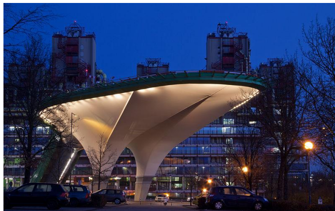
Figure 19 - Elevated Heliport Platform, University Hospital Aachen, Germany, [29].
