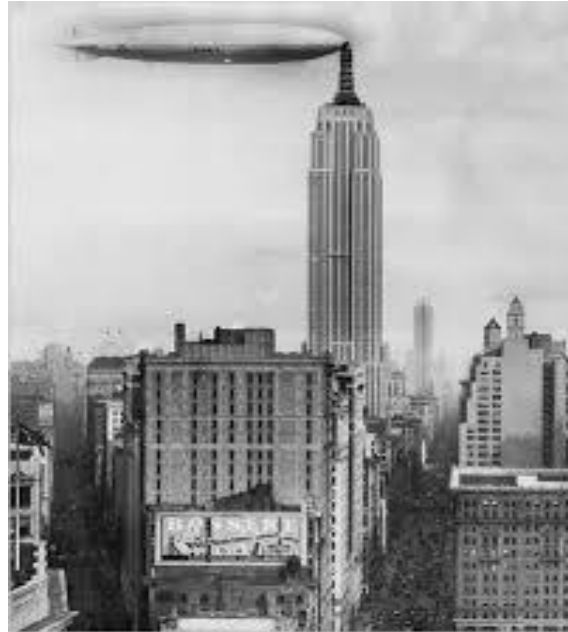
Figure 13 - Mooring Mast, Empire State Building, [27].
