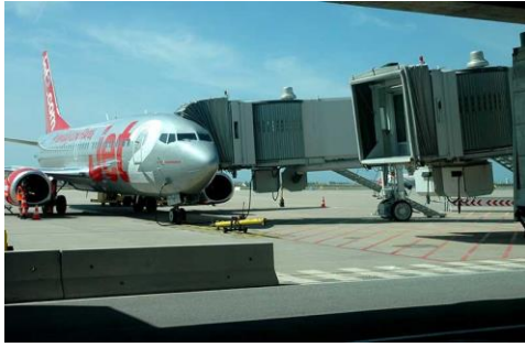
Figure 8: Airport boarding bridge (Trip Accessible, 2015)
