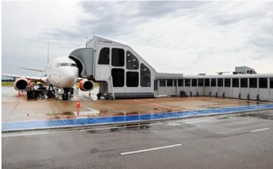
Figure 11: ELO system, a system of connectors (Infraero Aeroportos, 2014)
